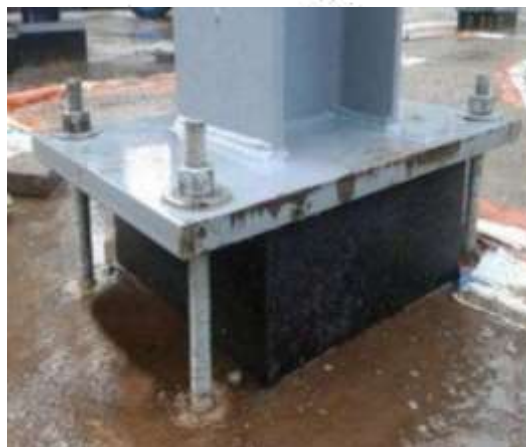
Fig 1 Elastomeric rubber bearing bridgesSliding Base Isolation Systems:
