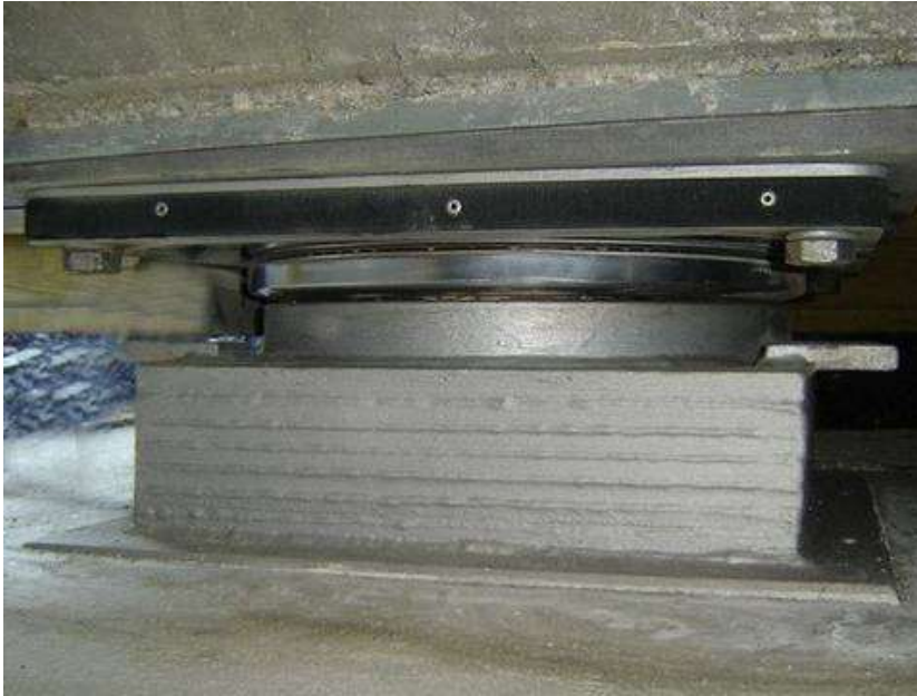
Fig 3 Spherical Sliding Base Isolation
