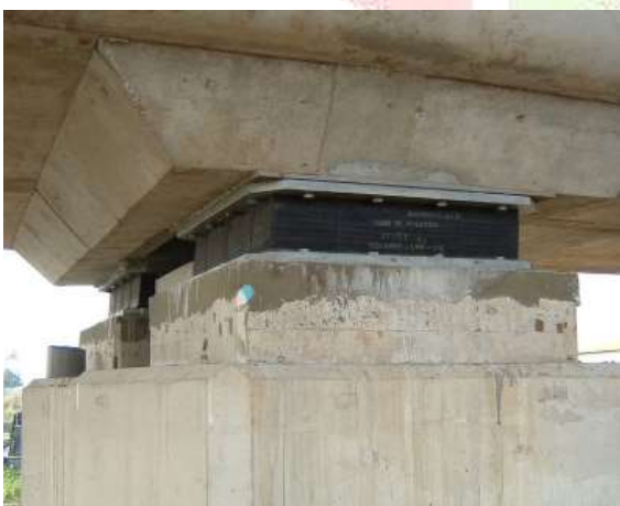
Fig 1 Elastomeric rubber bearing bridgesSliding Base Isolation Systems:
