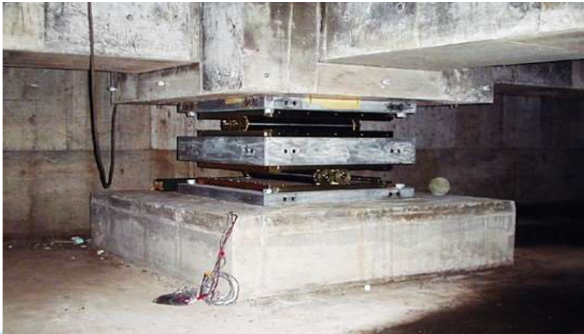
Fig 2 Sliding Base Isolation
