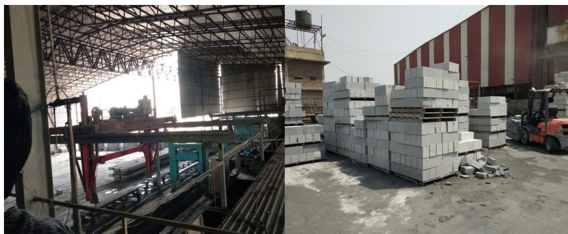
Figure 2: Plant view and AAC blocks
