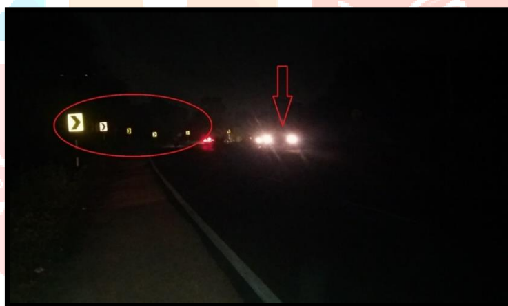
Fig 15 chevron sign boards illuminated at the curve.
