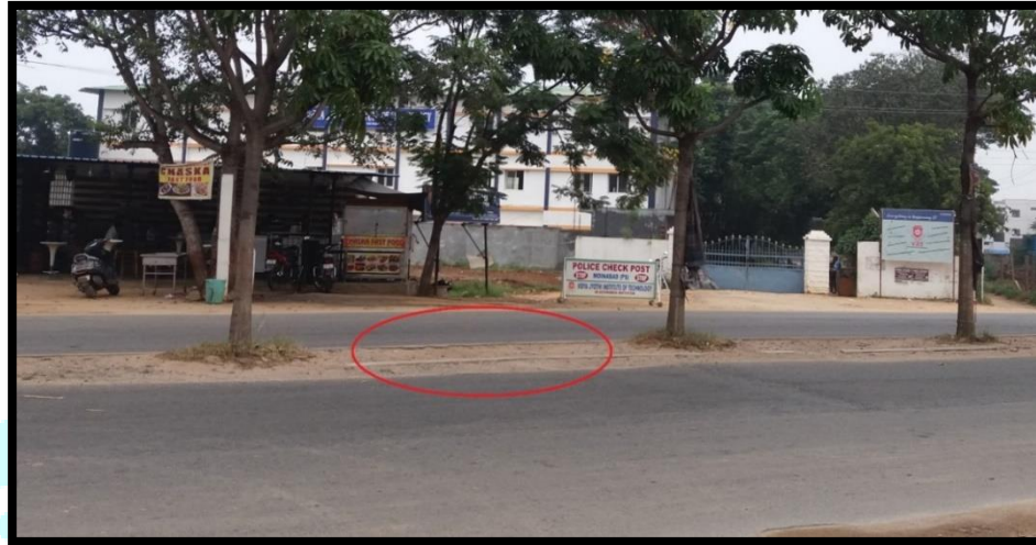
Fig 8 Median at the carriageway level.
