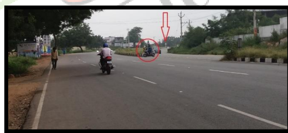
Fig 9 Median opening at the steep curve.
