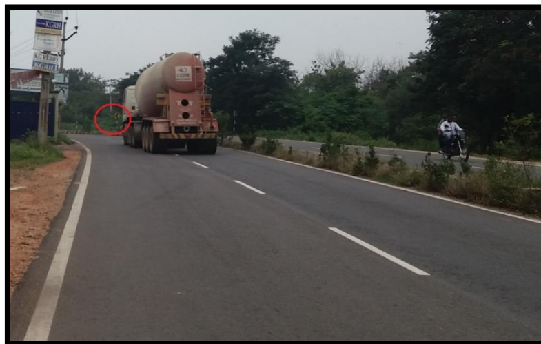
Fig 3 Horizontal curve clearly indicated by retroreflective Chevron signs.
