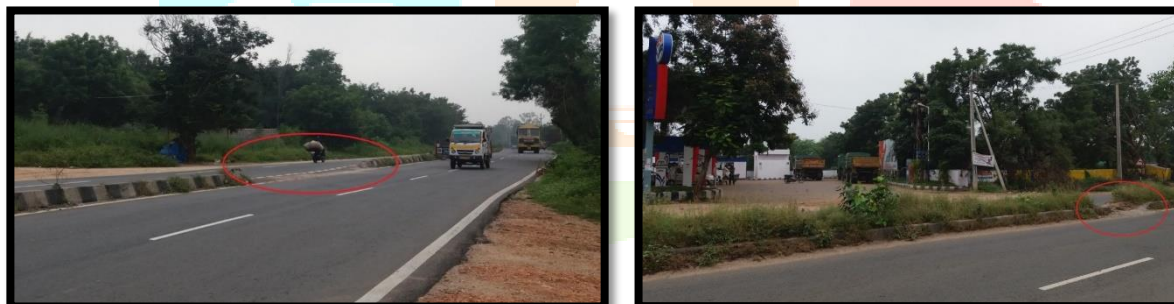
Fig 4 Illegal/ wrong/incorrect opening in the median.
