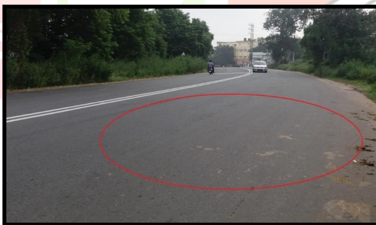
Fig 11 Absence of Super Elevation.
