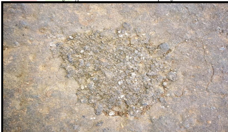
Fig.4 Pot Hole Repaired using WPA-Bitumen Mix.
