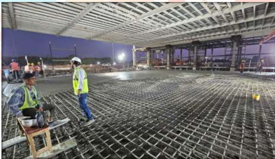
Fig.12. Above Precast slab 150 mm thk
