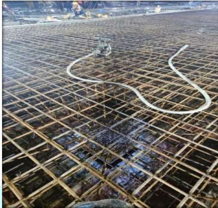
Fig.11. Cast in situ slab 700mm thk
