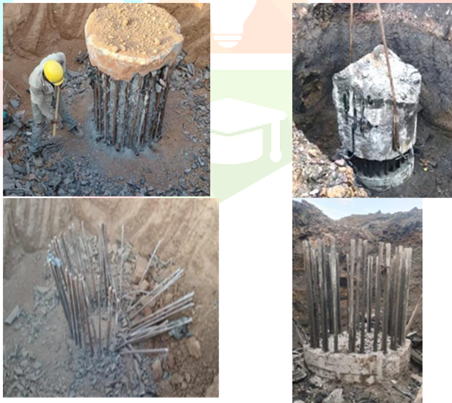
(a) Without Foam Sleeve (b) Concrete Detachment with Foam Sleeve (c) Exposed Concrete (d) Finished Look
