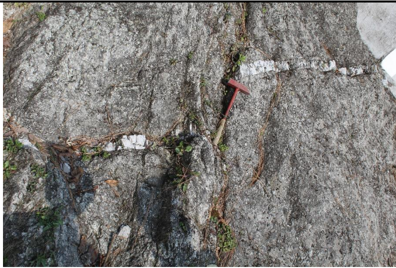
Fig. 5. Showing fault in granite
