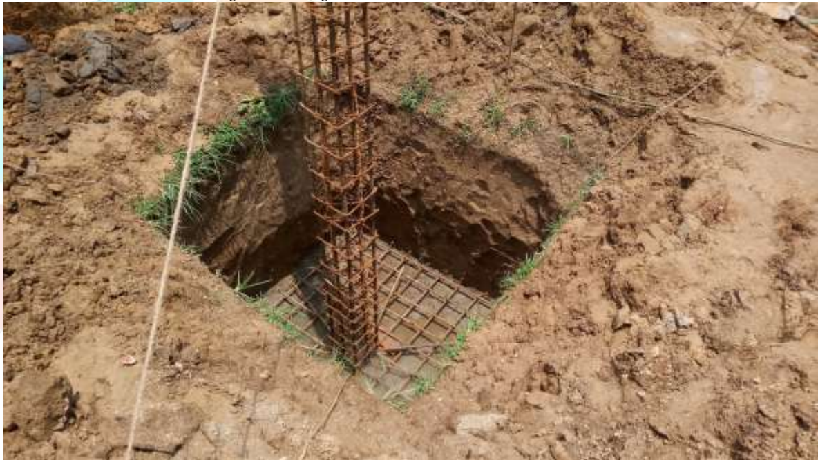
Fig: Foundation and Column Layout
