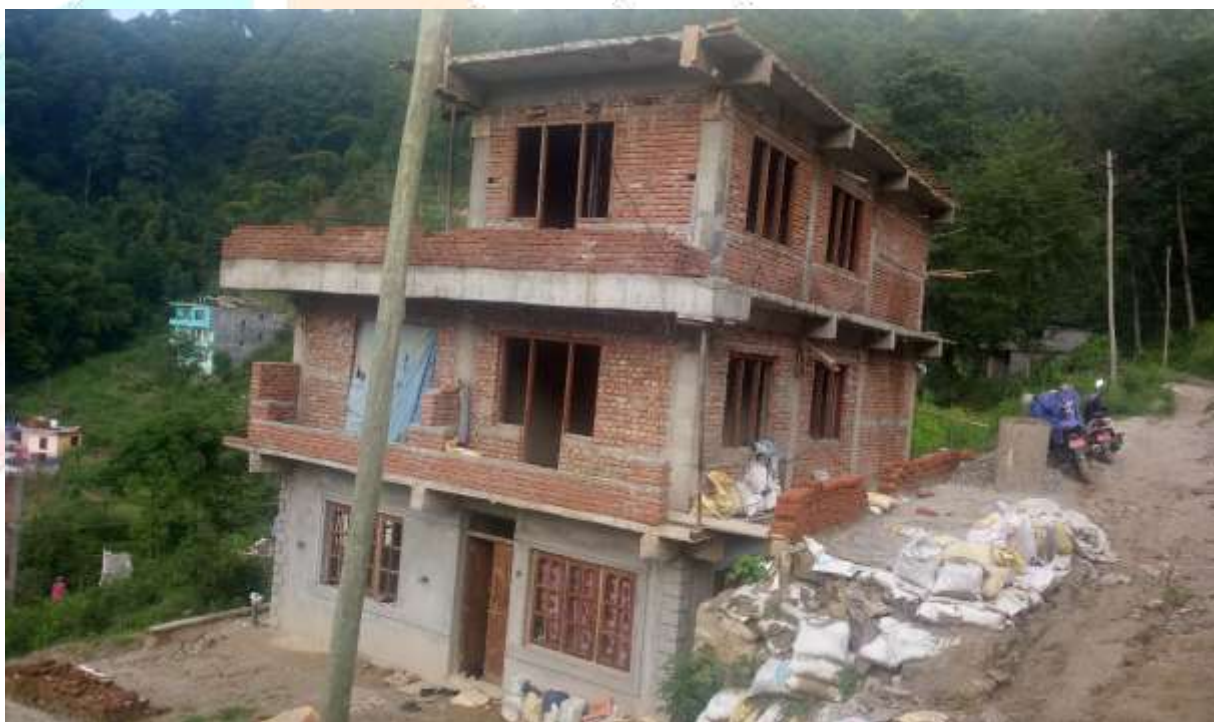
Fig: House under construction
