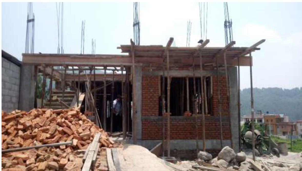
Fig: House under construction at Budhanilkantha
