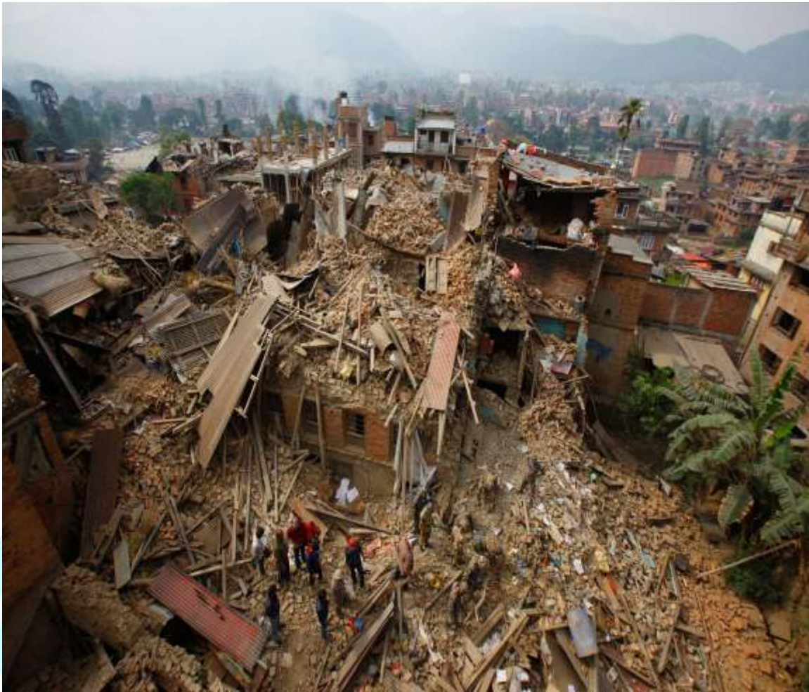
Fig 2: Destruction on Property due to Earthquake at Kathmandu Region
