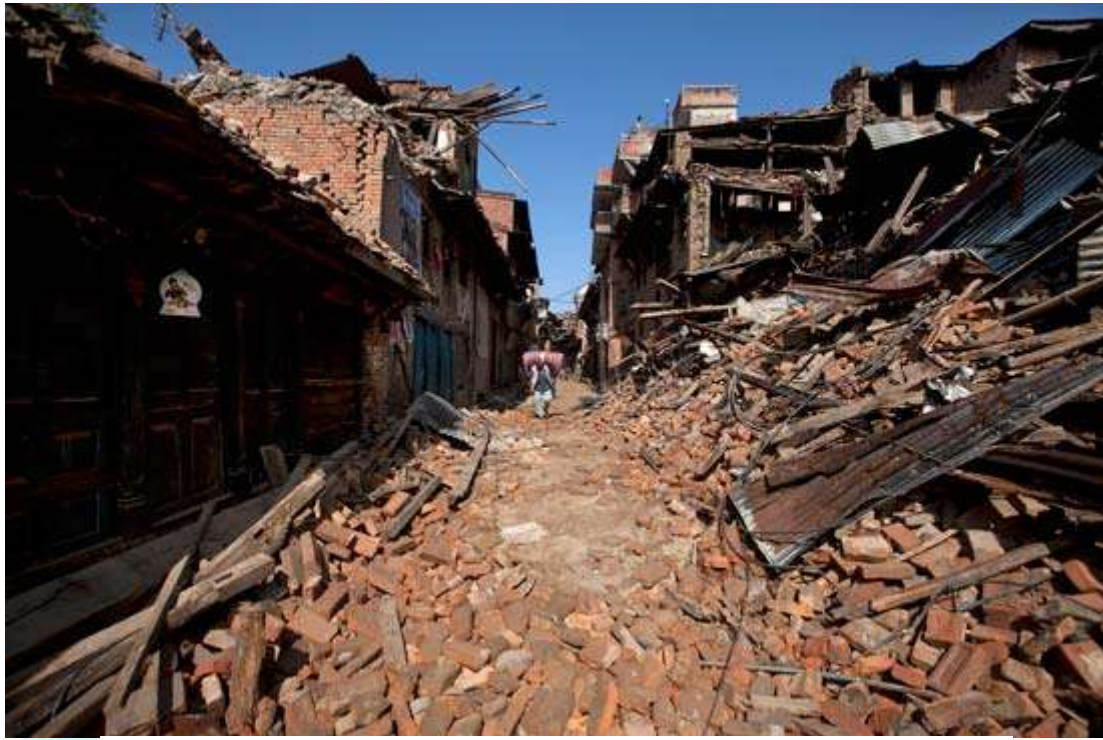
Fig 4: Destruction on Residential Buildings due to Earthquake at Kathmandu Region
