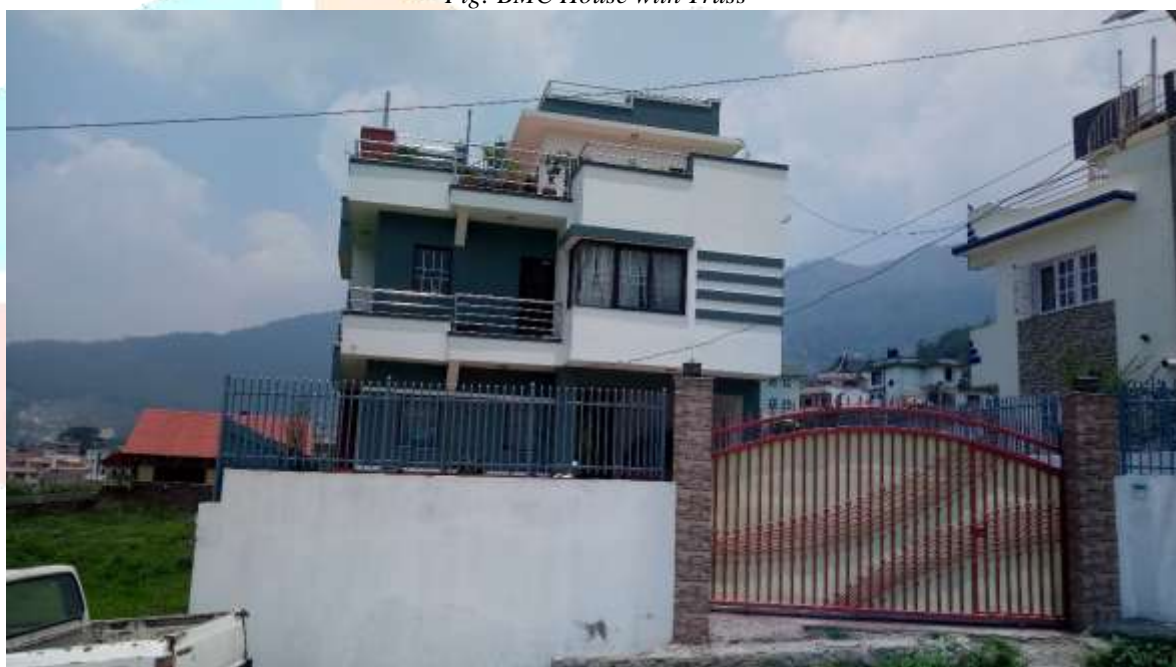
Fig: Recently constructed House
