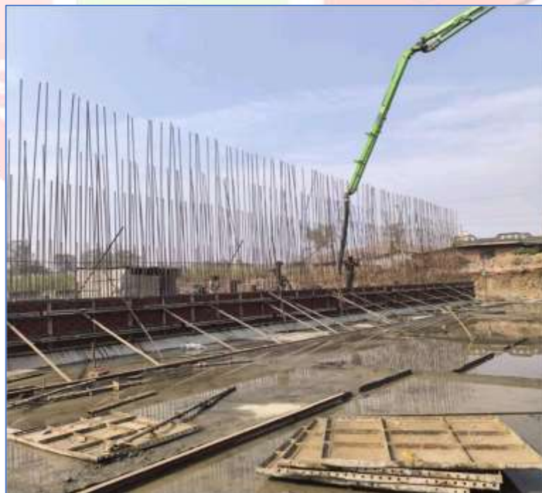
Fig. 2.4.2 Concrete of side wall
