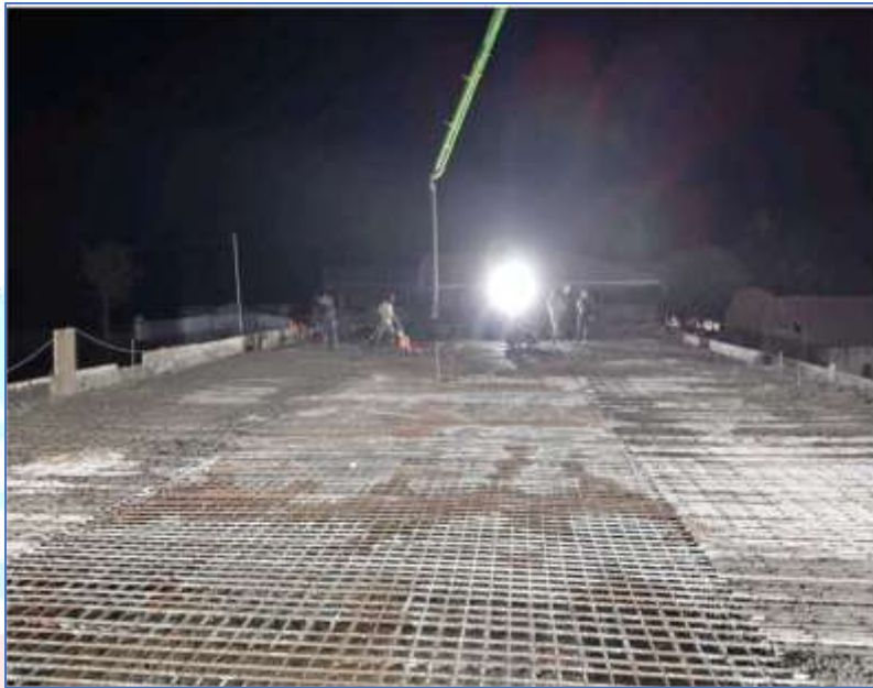
Fig. 2.5.2 Deck Slab Concrete work
