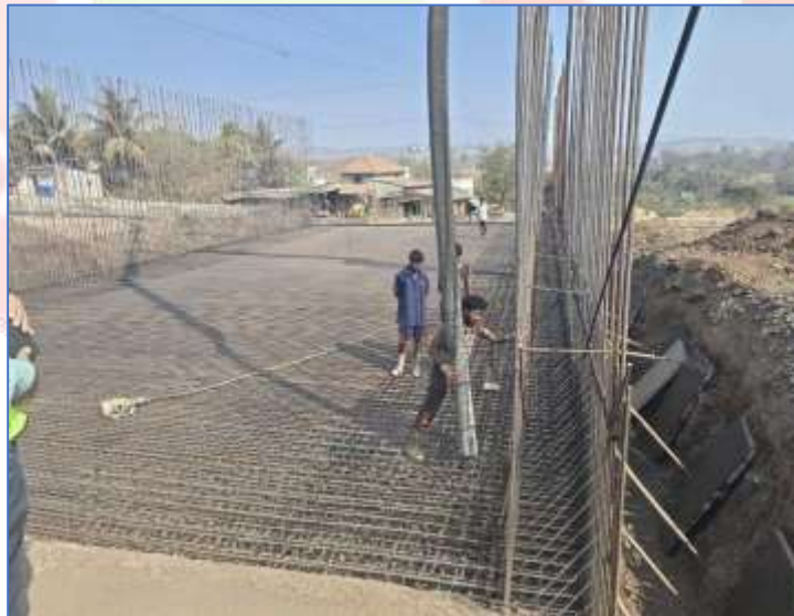
Fig. 2.3 Raft foundation Concrete work
