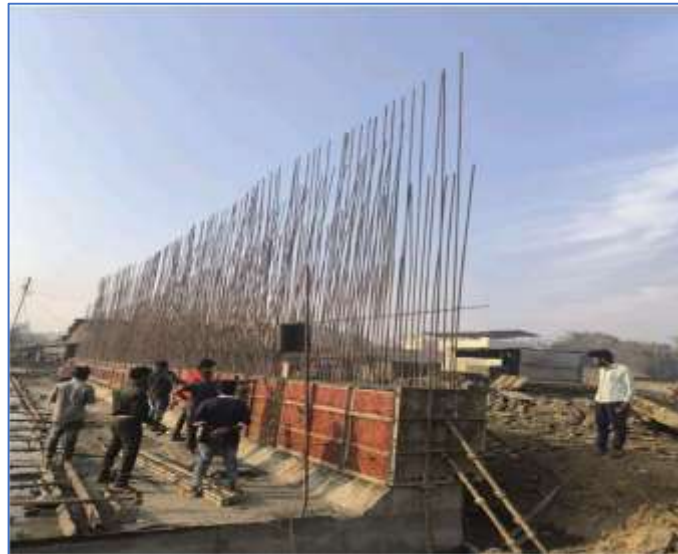
Fig.2.4.1 Shuttering of Side wall
