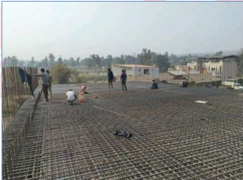
Fig. 2.5.1 Reinforcement of Deck Slab (LVUP)
