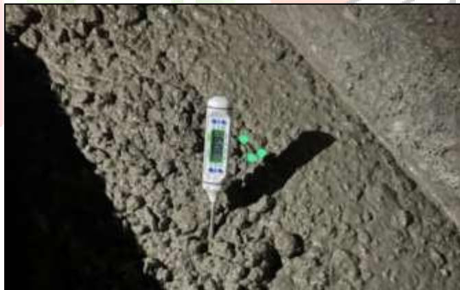
Fig.08. Concrete material (M45 Grade)
