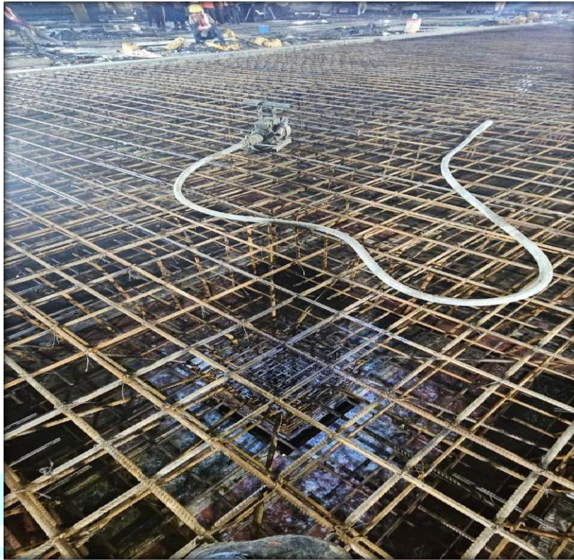
Fig.11. Cast in situ slab 700mm thk
