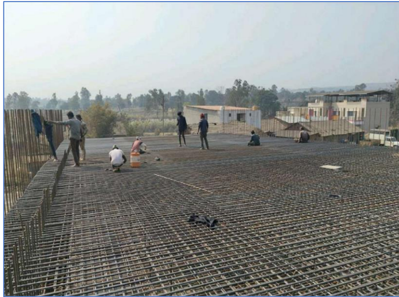
Fig. 2.5.1 Reinforcement of Deck Slab (LVUP)
