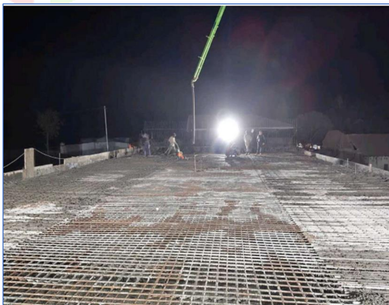
Fig. 2.5.2 Deck Slab Concrete work
