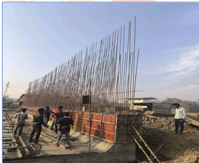
Fig.2.4.1 Shuttering of Side wall
