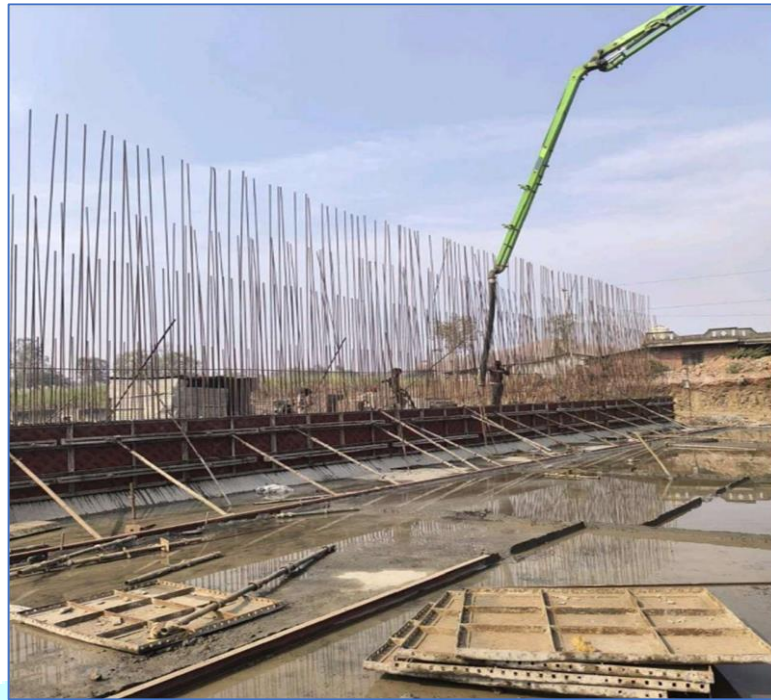
Fig. 2.4.2 Concrete of side wall
