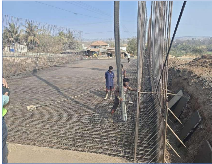
Fig. 2.3 Raft foundation Concrete work
