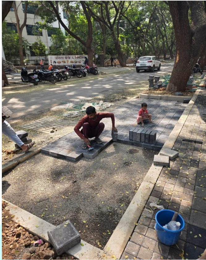
FIG. 4.2 PARKING PAVERS FIXING
