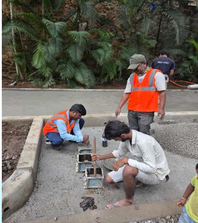
Fig.3.1.3. Concrete Cube filling
