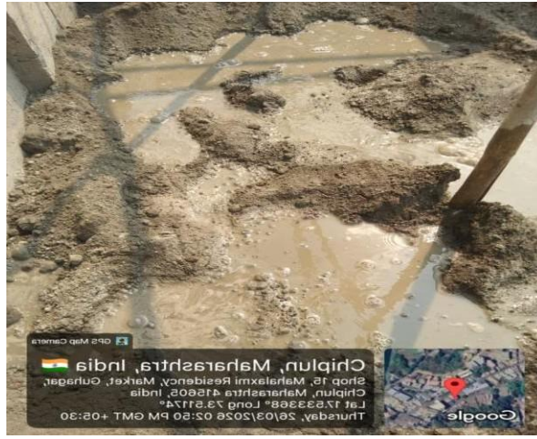
2. Fig of plaster mortar
