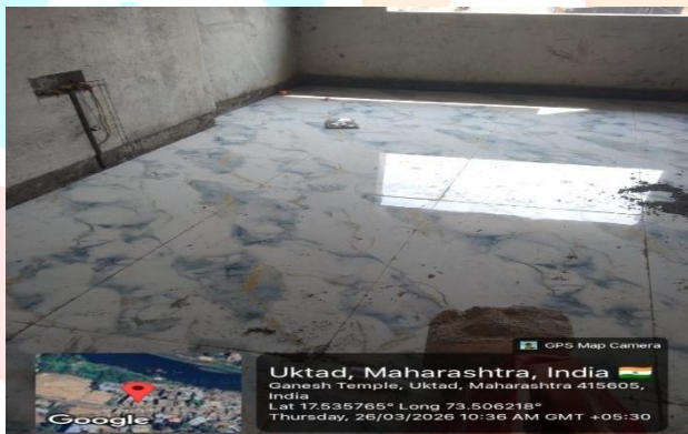
Fig.2.1 Completed Tile Flooring Surface
