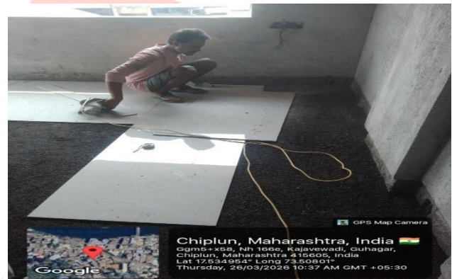
Fig. 2.2 Tile Placement in Progress
