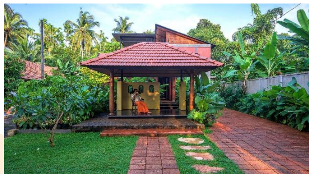
fig. 4.1.2. Entrance view of Chandroth residence
