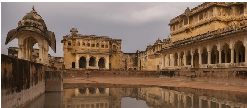
fig.4.3.1. Nagaur Fort View
