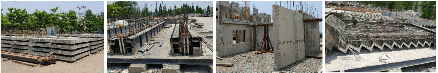
Fig. 10: PCC Construction Components – Precast Slabs, Precast Columns & Beams, Precast Wall Panels, Precast Staircases
