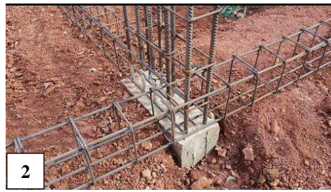
Fig. 4: Plinth Stage
