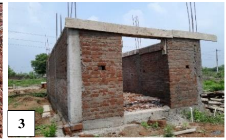
Fig. 5: Wall Construction Stage
