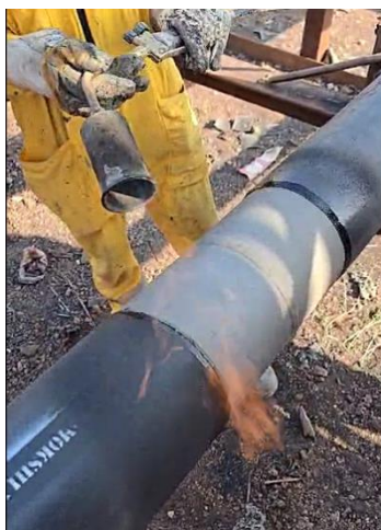
Fig 3.4 – Pipe Surface Drying by Heating Process and Drying
