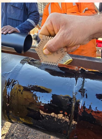
Fig 3.7 – Thickness Measure by Wet Film Thickness Gauge
