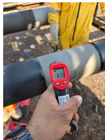
Fig 3.5 – Pipe Surface Temperature after Heating
