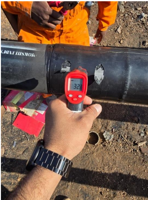
Fig 3.10 – Cooling Temp after Shrinking
