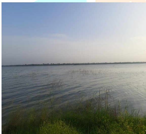
Fig.1. A view of Khaji kotnoor reservoir.
