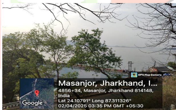
Fig.2:- View of Masanjore Dam Area
