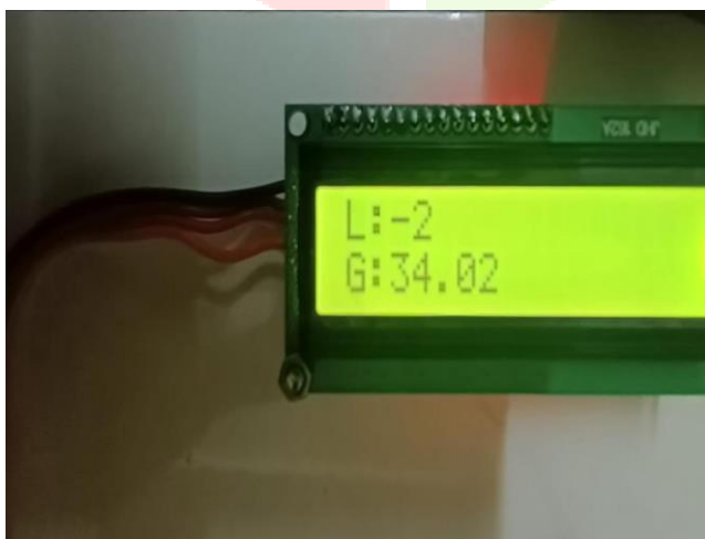
Fig 4. Real-time Gas Level and Leakage Status Display
