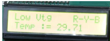
Figure 6. Under voltage fault detection on LCD display
