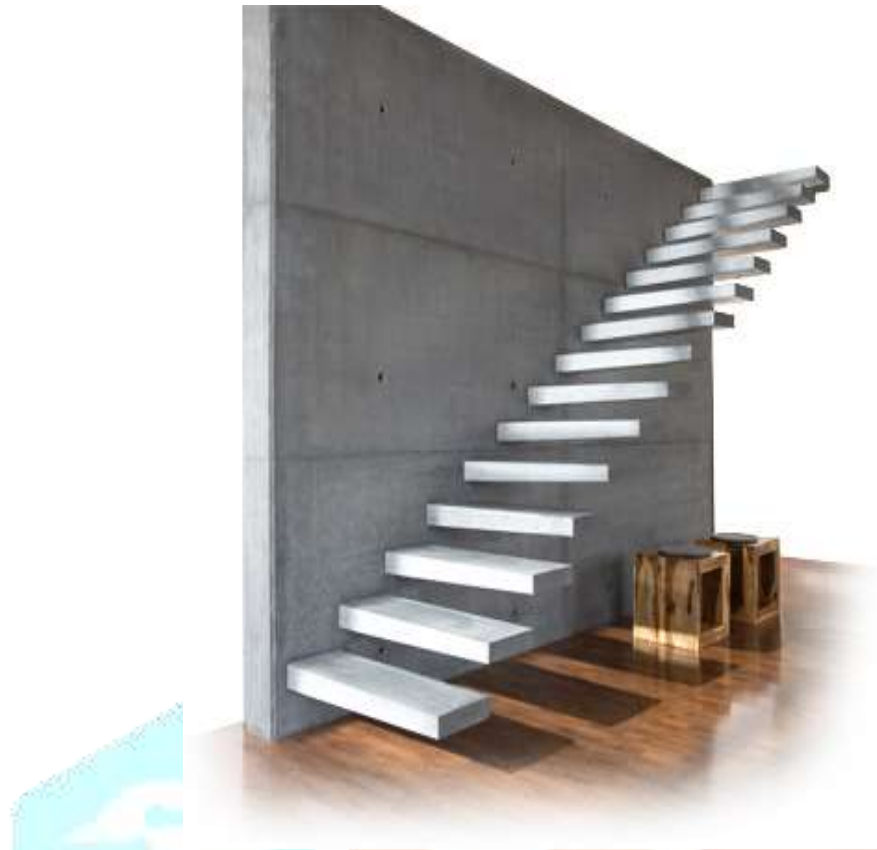
Fig. i) Stairs with cantilever steps that are supported on a shear wall
