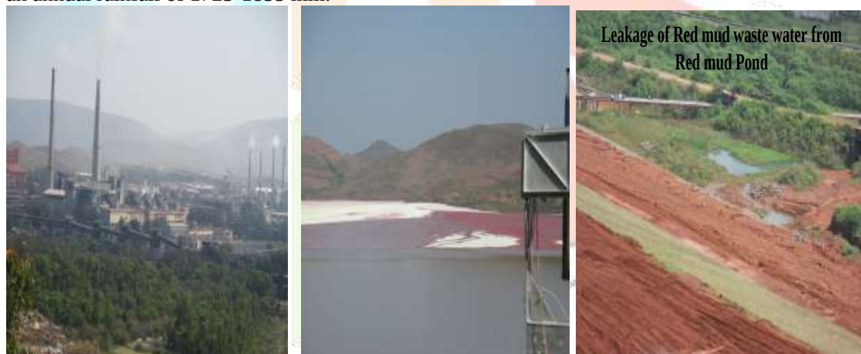
(P-1: The industry under study; P-2: Red mud Pond, P-3: Leachate leaking from the pond)
