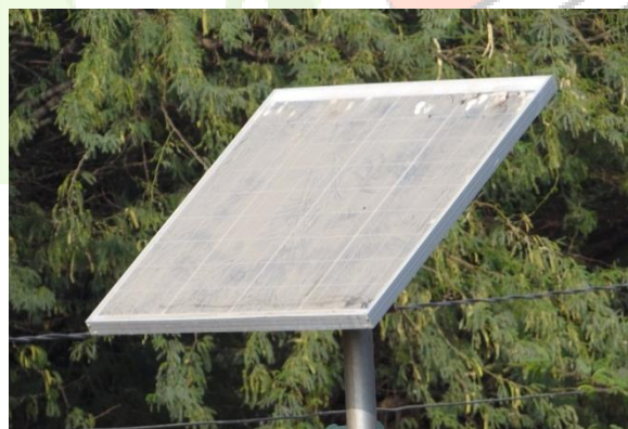
Fig. 1 Dust soiling on the solar photovoltaic plate at the height of 15 feet in an open environment.
