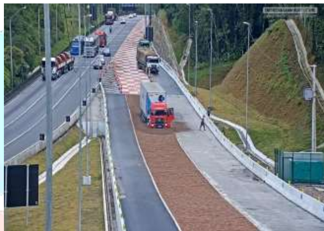
Figure 1. Emergency Escape Ramp
