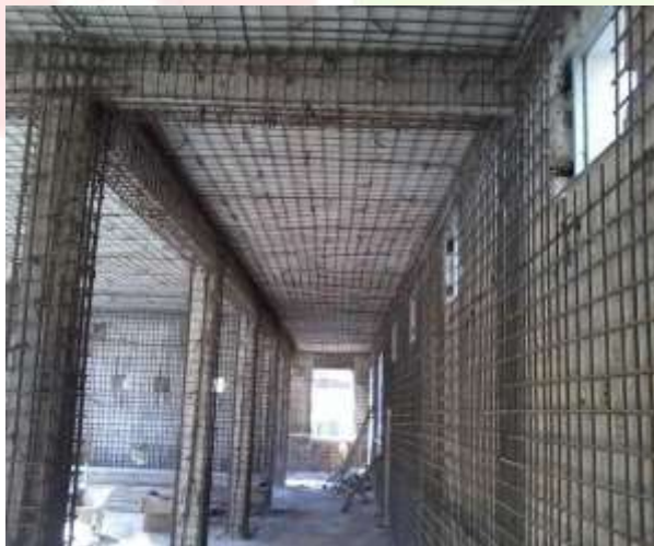
Fig 7. Details of Jacketing
