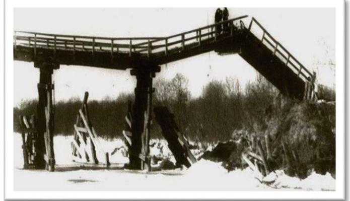
Buckling of bridge due to compression induced by earthquake
