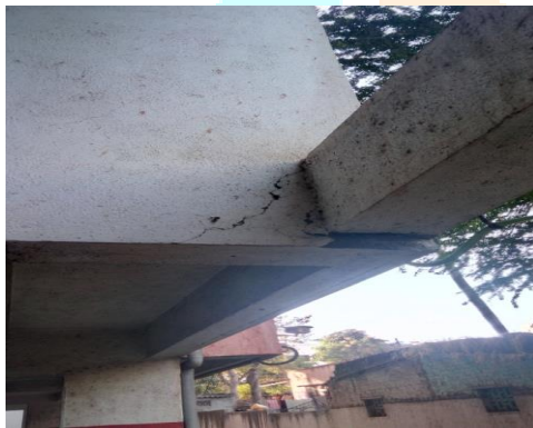
Fig. 5 - Diagonal cracks
