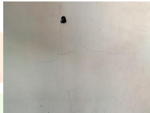
Fig. 6 - Hairline cracks
