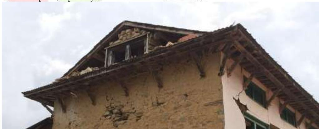
Figure 1 Gable End wall Collapse
