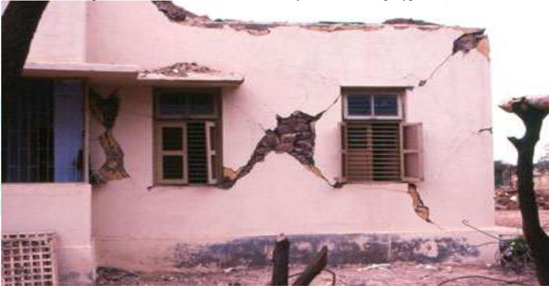
*Figure 1 In-Plane Failure*
